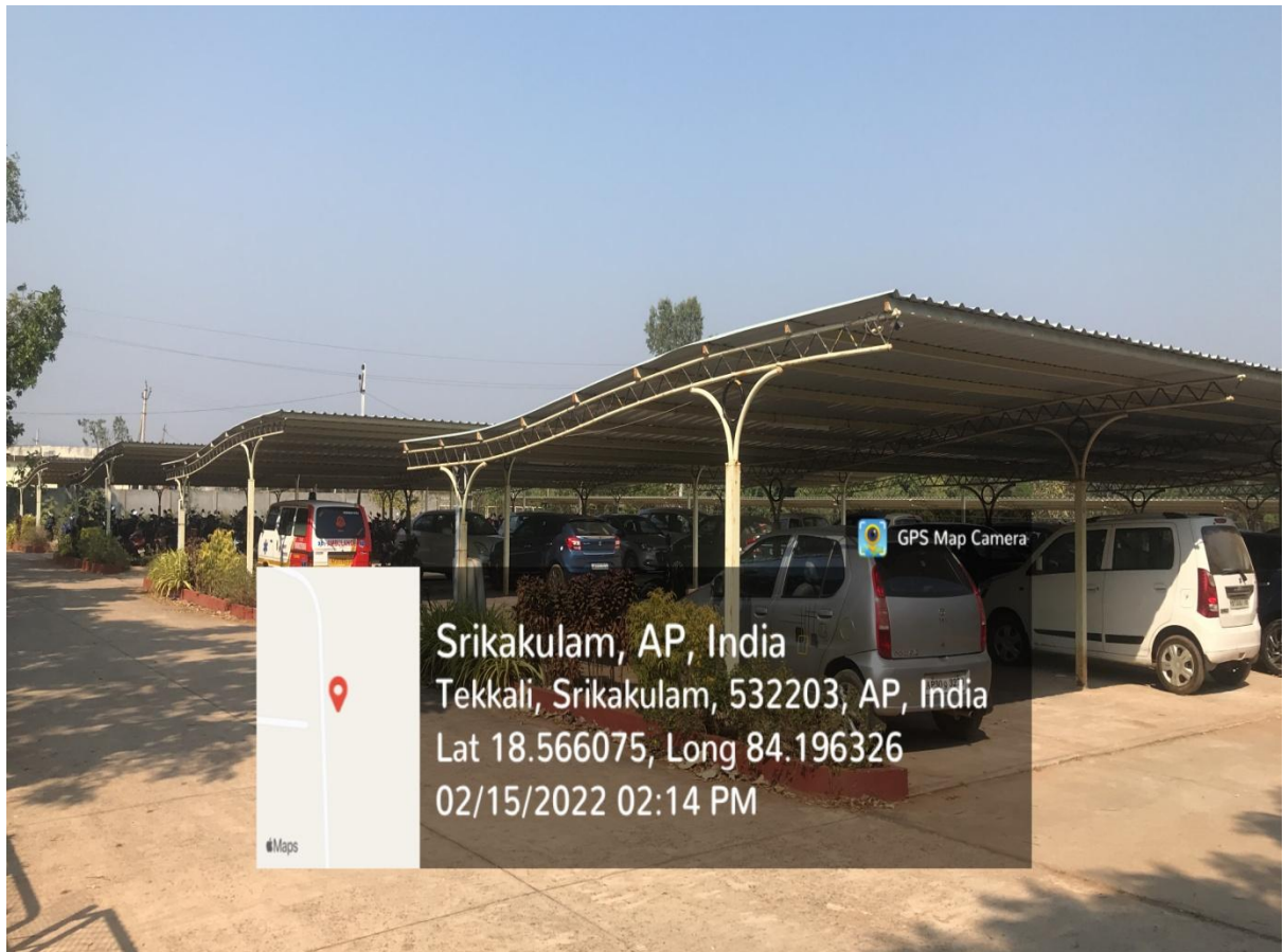
Central Parking Area
